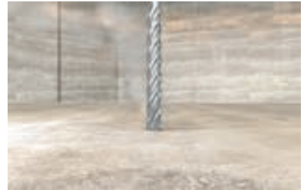
Bohren in Bodenplatte
